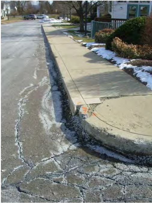
1. Cracking and spalling walks, paving cracking
