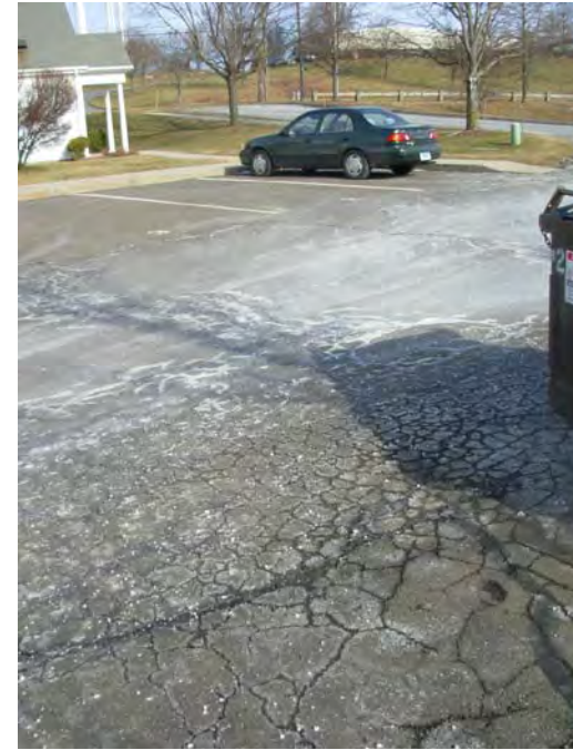
2. Cracking and settlement of asphalt paving
