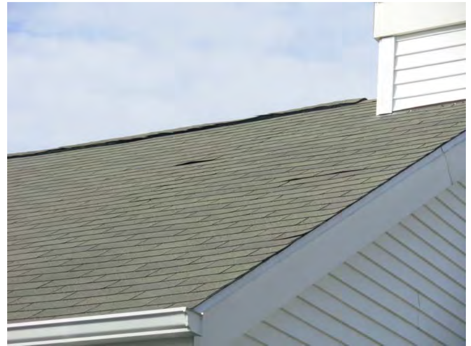
10. Spot lifting of roofing shingles
