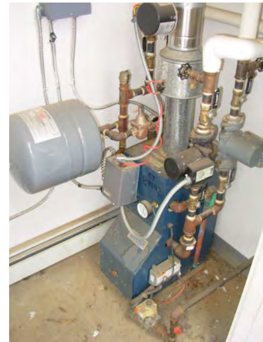
16. Typical unit heating boilers and peripherals
