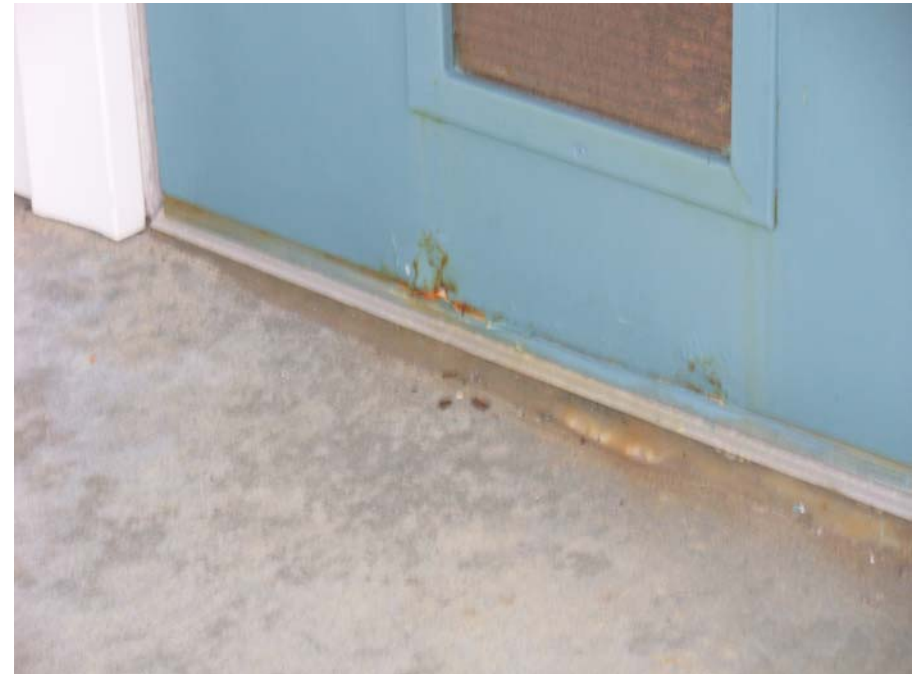
8. Spot rusting of service and unit doors
