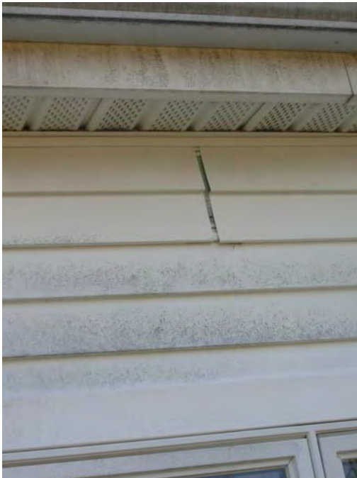
7. Spot vinyl siding seam separation, organic growth
